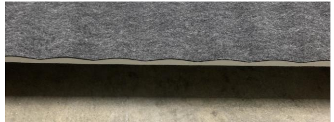
Side view of panel suspended by 50 mm prior to skirt installation
