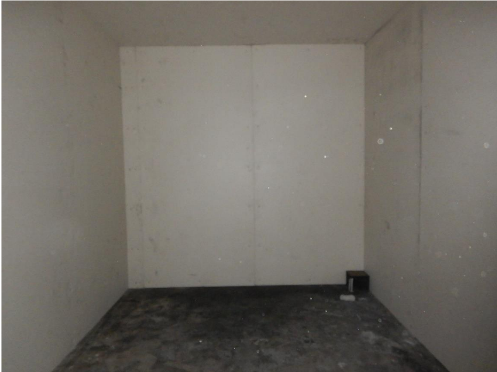
Figure A4.1. Exposed corner of the specimen before commencement of the reaction to fire test.
