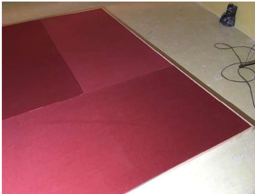
Figure 3: 25mm absorption panels with an mdf perimeter
